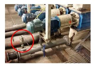
The admixture of lime during the flue gas cleaning is realized with different conveying systems. The already described conveying system with the use of a conveying screw is an exception, more common is the transportation by an airstream. Thereby the lime is admixed with the help of a rotary feeder, the amount of lime is constant and it is not regulated. In this case the SolidFlow transmits the measured quantity to a control room to control and display it.
