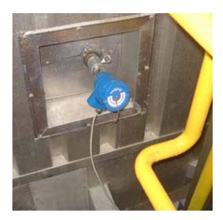
Reliable and safe dust measurement on the clean side oft he baghouse filter, generation of a reliable and continuous absolute value.
